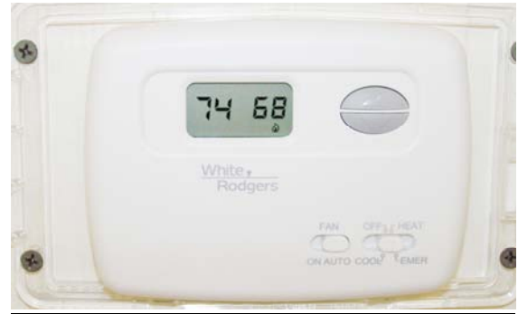
Heat Pump, Switch Set to Position 3
