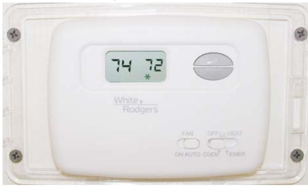
Air Condition On, Switch Set to Position 2
